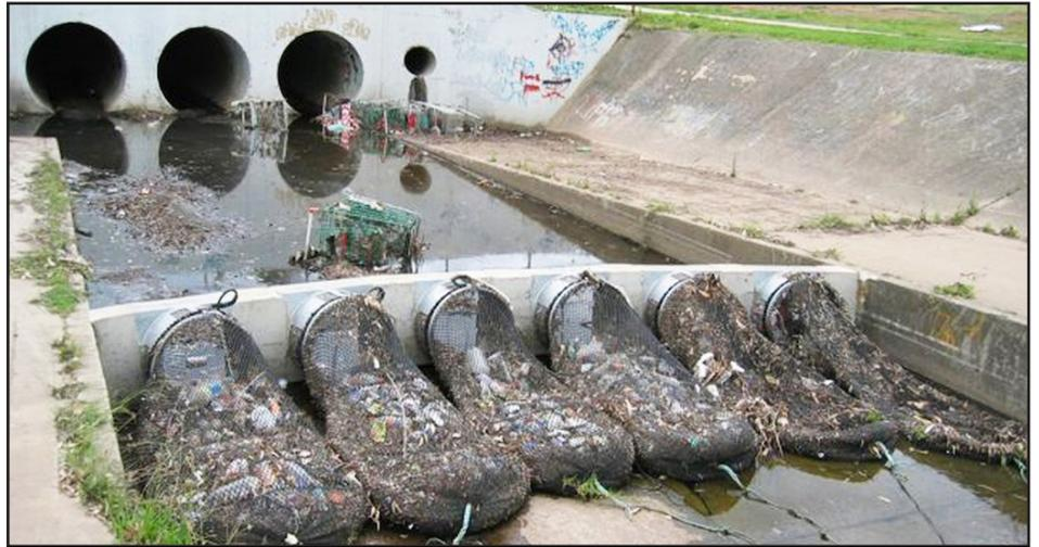
A series of nets used in a storm drain system in California to prevent trash from reaching local streams and the coast. Photo credit: Stormwater Systems, Inc.
