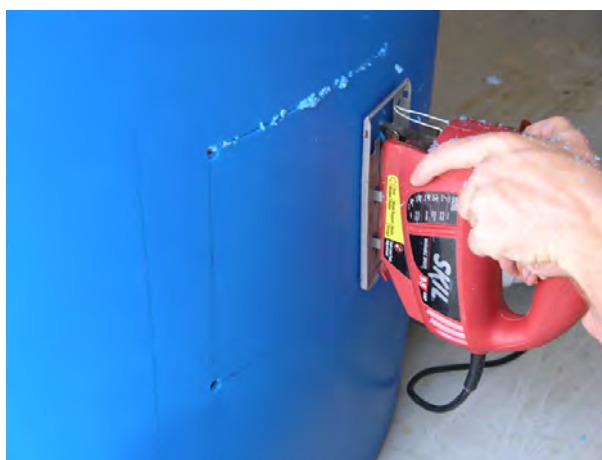
Figure 19. Continue cutting with the jigsaw until the space for the window is cut out
