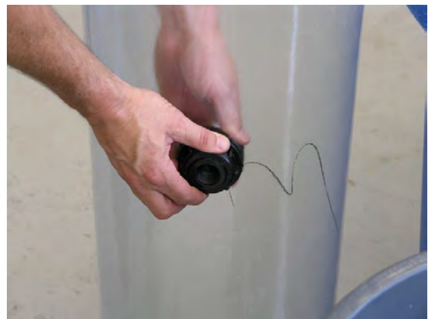
Figure 13. Thread a 3/4" bulkhead into the biofilter using the SBP
