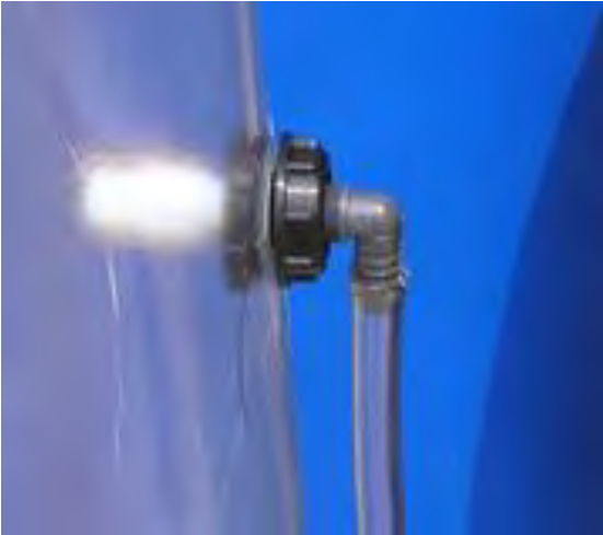
Figure 14. Rotate the male 90° ell so that it points straight down
