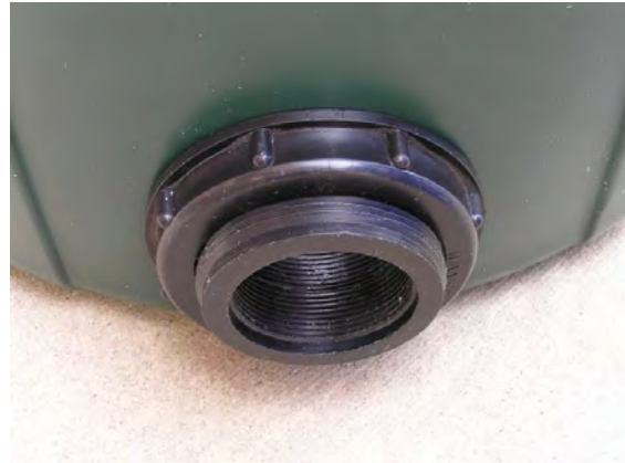
Figure 6. Using the SBP, place a 2" bulkhead into trash can/sump
