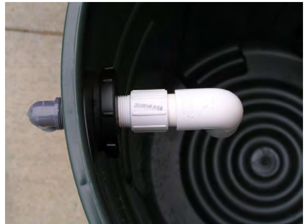
Figure 10. The internal plumbing draws water from below the sump's surface
