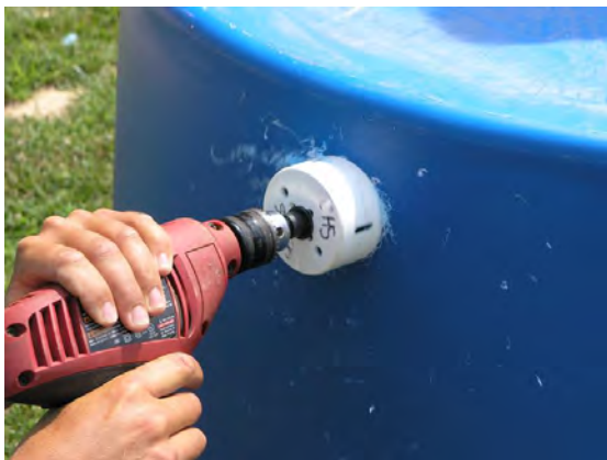
Figure 3. Cut a hole for the 2" bulkhead
