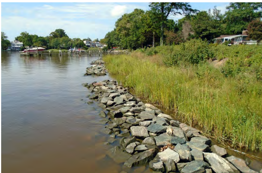
Living shoreline in Maryland. Photo, Eric Buehl, University of Maryland Sea Grant Extension
