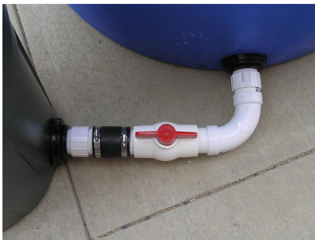
Figure 7. The completed plumbing assembly allows water to move from tank to pump
