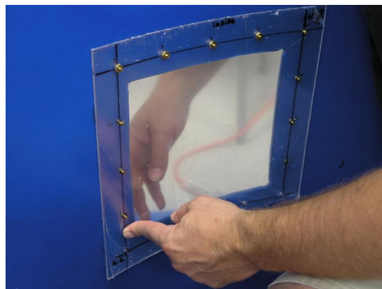
Figure 21. Do a trial fit of the window without gluing
