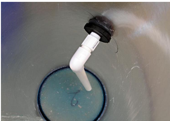
Figure 15. Since this piece is entirely internal and leakage is not a concern, you do not need to use Teflon tape or pipe dope
