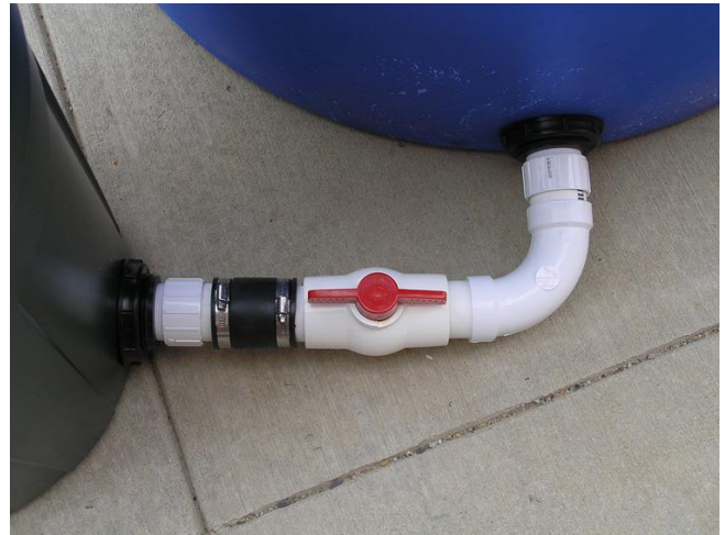
Figure 7. The completed plumbing assembly allows water to move from tank to pump
