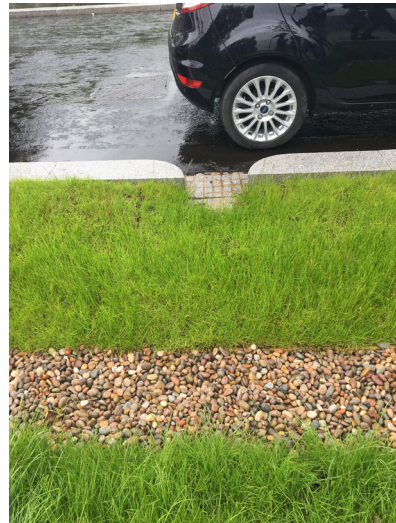
Example of a stormwater retrofit in the Clyde Gateway community in Glasgow, Scotland. Image: Jennifer Dindinger
