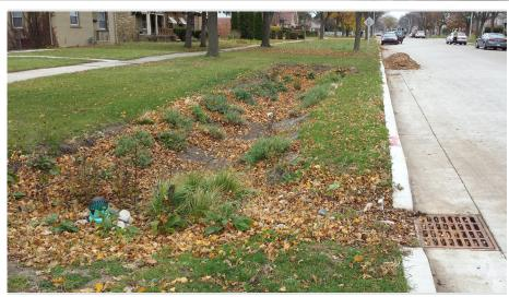
Along with the installation of several large stormwater management basins in the 30th Street Corridor in north central Milwaukee, MMSD is using dispersed green infrastructure practices such as this street-side bioretention facility which will help to decrease the volume of stormwater runoff they need to capture and treat. Source: Eric Buehl
