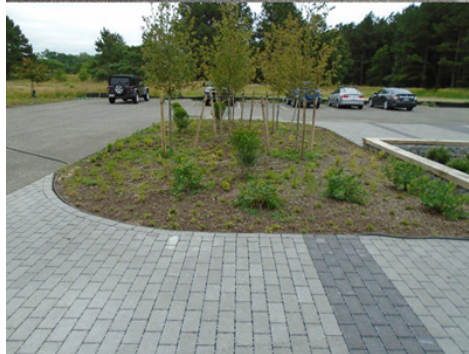
Before image top/After image bottom: Despite their best efforts, keeping plants alive in this parking island was difficult. Now it's part of the stormwater system and helps to decrease runoff and will eventually provide shade when the trees get taller. Source: Eric Buehl.
