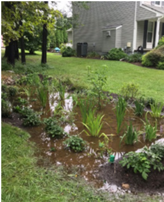
GI rain garden at work in a 1 inch rainstorm. Source: A. Rockler
