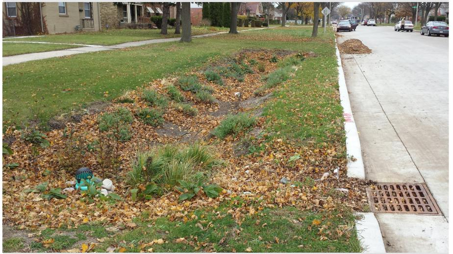
Along with the installation of several large stormwater management basins in the 30th Street Corridor in north central Milwaukee, MMSD is using dispersed green infrastructure practices such as this street-side bioretention facility which will help to decrease the volume of stormwater runoff they need to capture and treat. Source: Eric Buehl
