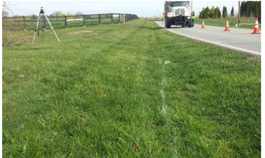
The roadside ditch before installation. Photo Credit: Eric Buehl
