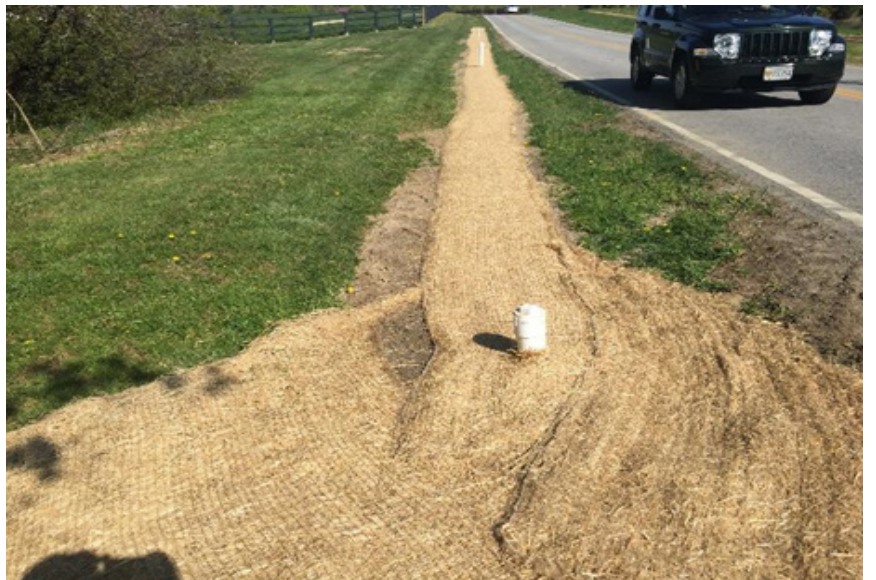
The roadside ditch after installation. Photo Credit: Marshall McSorley
