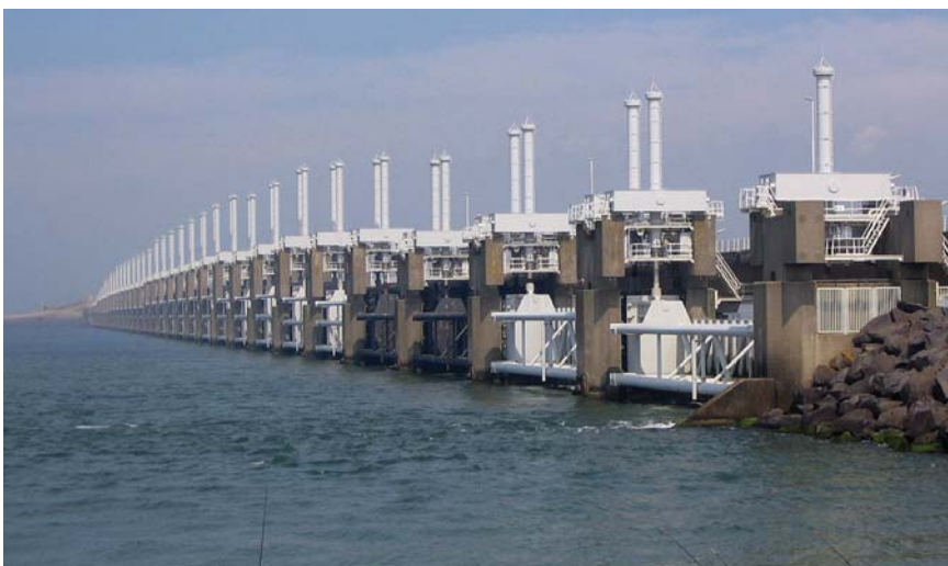
The disastrous North Sea Flood of 1953 spurred the government of the Netherlands to start work on the Deltaworks Project, a series of dams, dikes, sluices, locks, and levees to protect against another catastrophic storm surge. The Oosterscheldekering storm surge barrier (shown above) is the largest structure in the system, stretching nine kilometers and including sluice gates that are only closed during flood threats. PHOTO, VLADIMIR ŠIMAN
