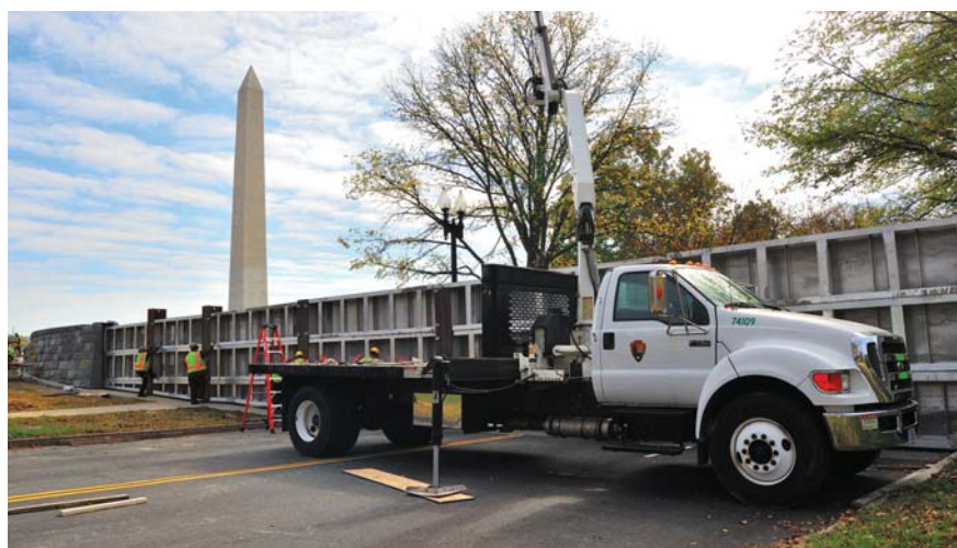
Rolando Sanidad, project manager for the U.S. Army Corps of Engineers (top), stands by the east stone wall, one of two permanent pieces of the flood wall to block off 17th Street during major flood events. The removable panels of the flood wall connect to the west stone wall on the other side of the street. With posts and panels finally in place, the removable flood wall puts a nine-foot barrier between downtown D.C. and the Potomac River (bottom). PHOTOS, MICHAEL W. FINCHAM
