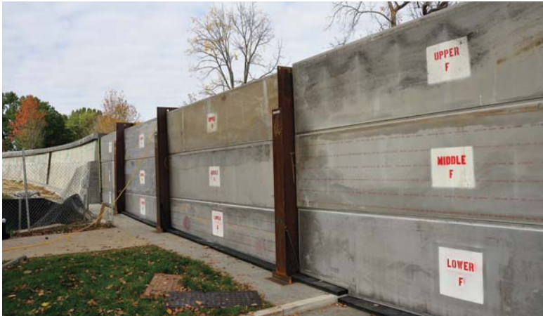
An artist's sketch shows an early version of the 17th-Street flood wall (top). The photo below shows the "post-and-panel" flood wall with labeled panels in place during the test assembly on Halloween 2014. The Washington wall has nine posts and 27 panels, all of them stored off-site. When a major flood event threatens the city, they will be trucked to 17th Street and craned into place. DRAWING, COURTESY OF THE U.S. ARMY CORPS OF ENGINEERS; PHOTO, MICHAEL W. FINCHAM
