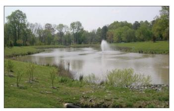
Stormwater ponds, like this one in Easton, Maryland, capture runoff and reduce nutrients in the water.
